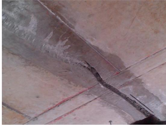
The active crystal slurry is applied as base coat before application of supportive specific repair mortar.
