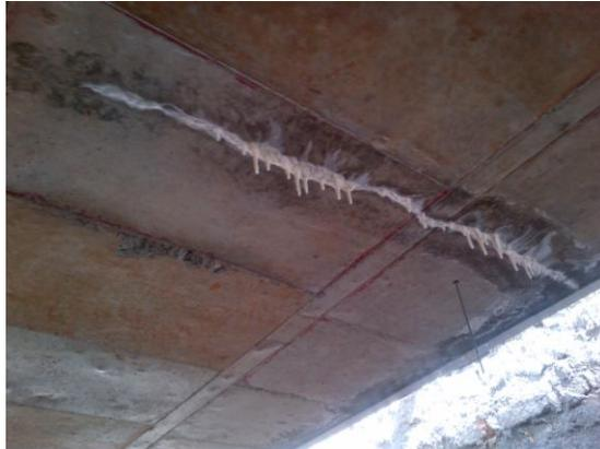
The still actively leaking crack is chased for preparation before the two stage product application.
