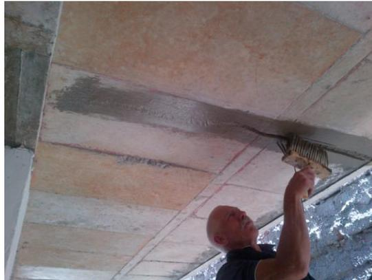
Specialized repair mortar is then applied to the chased section. I want to draw your attention the amount of water still seeping through the slab to the left of the image where the repair area was not chased, but merely coated with the active crystal slurry which is already diminishing.
