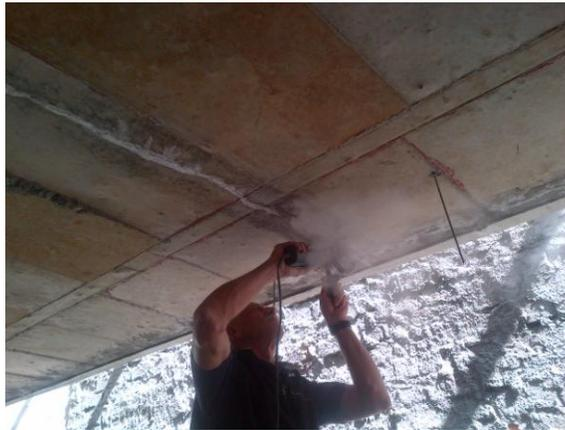
Chased area cleaned and “polished” before the next step in the process. Note how wet the prepared sections still are from the water that is still actively seeping through the crack.
