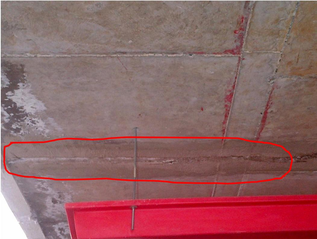
The section merely painted with the active crystal slurry is already 90% dry and will be 100% dry in the next few days once the crystals have sufficiently grown inside the crack in the slab.
